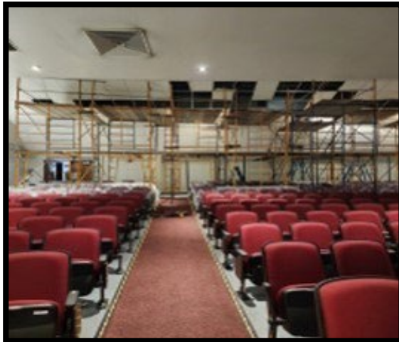
Typical Scaffold Set-Up
