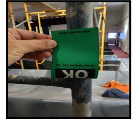
Inspection Tag Shows No Evidence of Inspection Prior to Use An OSHA Requirement Improvement needed
