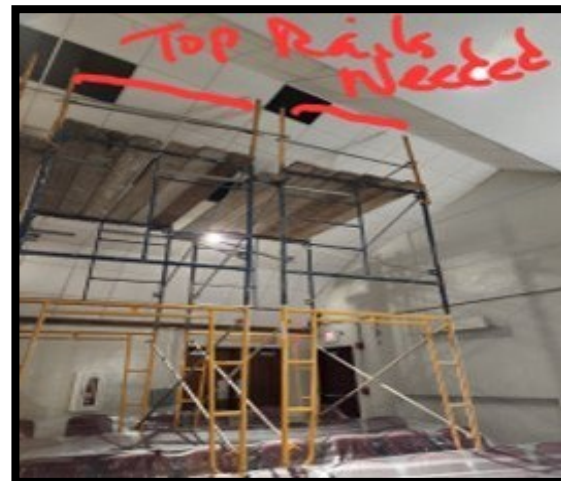
Working level-missing top rail
